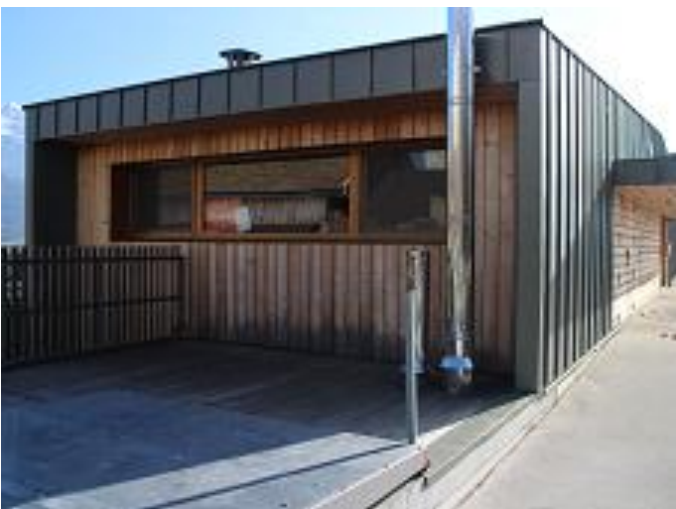
la chaufferie collective
